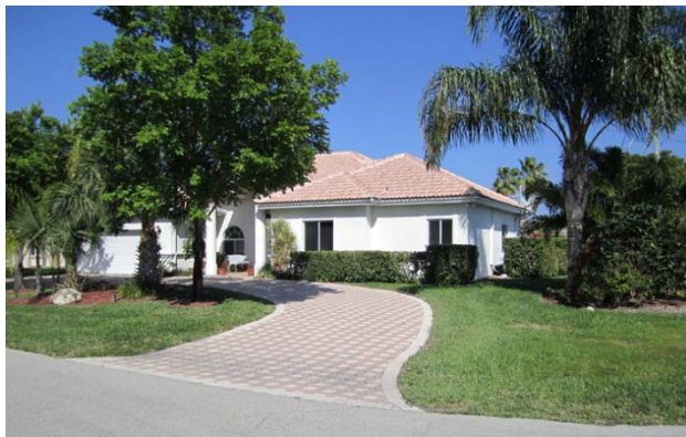
Example of a well maintained single family home
