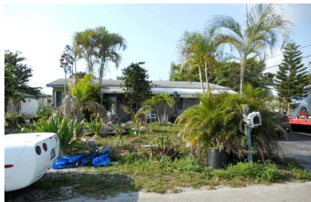
Example of a poorly maintained home with several code violations
